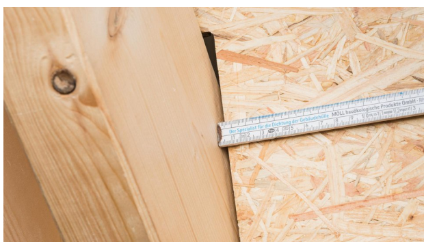
3. Check the joint width
