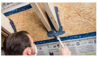
8. Check the joint If necessary, seal any gaps with a brush and AEROSANA VISCONN / FIBRE.
