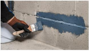
**5. Filling cracks up to 20 mm (0.8") in width** For cracks of 8 - 20 mm (0.3"- 0.8") in width, apply AEROSANA VISCONN FIBRE deep into the crack. To do so, the gap must be filled with sealant to a depth of at least half the width of the gap.
