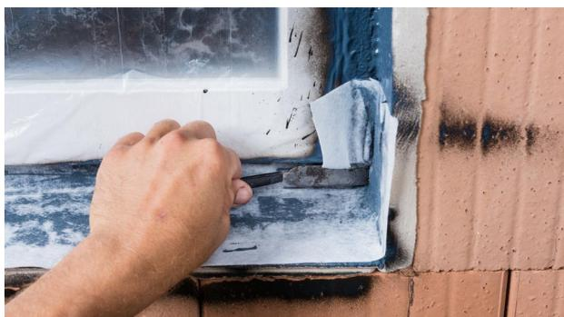
**7. Install the AEROSANA FLEECE sub-sill flashing**
