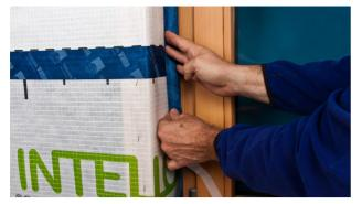
4. Stick the tape in place around the circumference of the soffit
