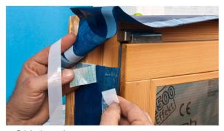
**3. Stick the ends** To ensure proper airtightness and/or wind sealing, stick the start and end of the CONTEGA IQ tape to each other using a strip of DUPLEX.
