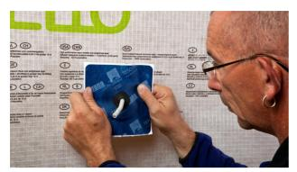
**1. Pull the cable through and align** Pull the cable through the pre-punched hole in the EPDM, guide the grommet as far as the subsurface and align. Suitable for cables with a diameter of 4.8 - 12 mm (3/16"-1/2").
