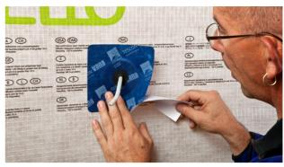
**2. Remove the release film** Gradually remove the release film.
