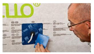
**3. Stick the grommet and rub it firmly in place** Stick the grommet to the subsurface and rub it firmly in place.
