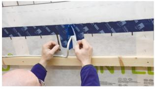
**5. Remove the remaining release film** Finally, remove all of the release paper strips at the folded flaps
