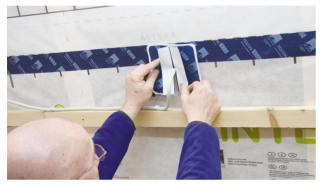
**3. Align the grommet** Guide the grommet with the slit around the cable and align it.
