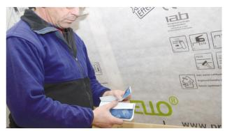
**2. Open the grommet at the slit** KAFLEX post has a slit and punched opening for the cable to be sealed. Gently pull the grommet apart at the slit.
