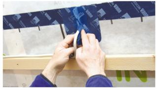
**6. Rub onto the cable** Stick the folded flaps to one another and to the cable in an airtight manner, and rub firmly in place. Ensure there is good adhesion in the corners. You're finished!
