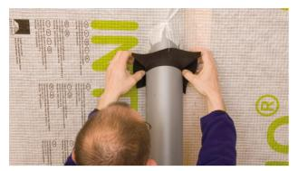
**1. Pull the grommet over the pipe and align it** Select a grommet to match the diameter of the pipe, pull it over the pipe, guide it as far as the subsurface and align it.
