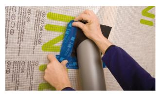
2. Stick the grommet and rub it firmly in place Stick the grommet to the subsurface and rub it firmly in place. Ensure that there is sufficient resistance pressure. This work can be carried out more efficiently and in a manner that is kinder to your hands by using the pro clima PRESSFIX application tool.
