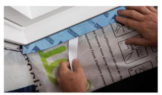
**2. Stick the second independent adhesive strip** Then remove the release film and gradually stick the tape to the second surface (in this case, onto the window reveal).
