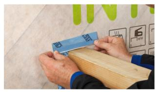
**5. Bonding with a narrow independent adhesive strip** The tape with a 12/38 mm split is ideal for bonding to components that will subsequently be covered only by a thin layer, e.g. with plasterboard.
