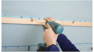
**9a. Detail solution for blown-in insulation material** If blown-in insulation material is to be used, secure the overlap taping with a supporting lath. Use suitable vapour check membranes (e.g. DB+).
