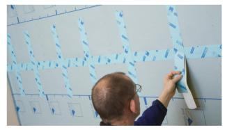
**9b. Detail solution for blown-in insulation material** Alternative: under certain conditions, the use of perpendicular support strips of tape at maximum intervals of 30 cm (12") may be sufficient. It is your responsibility to verify this on site.
