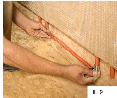
*When bending the pipes, observe a minimum bending radius of 80 mm, when bending by hand, and of 64 mm, when using a spiral spring!*
